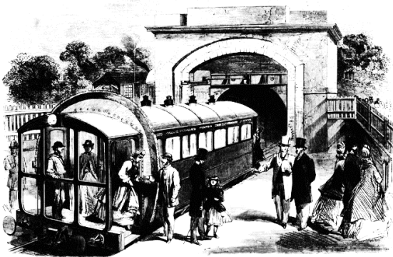
Above: Thomas Rammell's railway at Sydenham. A carriage with a large collar of bristles was sucked along an air-tight tunnel.
